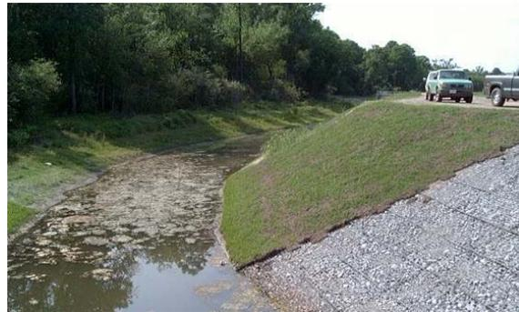
The view on the left (above) shows the soil lifts and Mirafi Geogrid which wrapped the lifts. The right photo shows the area at final project acceptance, with gabion baskets adjacent to the flow diversion structure into Lake Henrietta.
