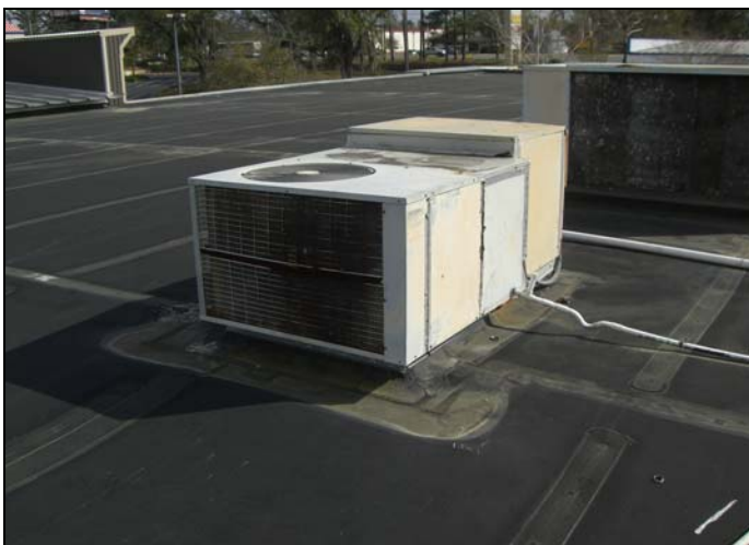
Building Roofing Repairs and Replacement
