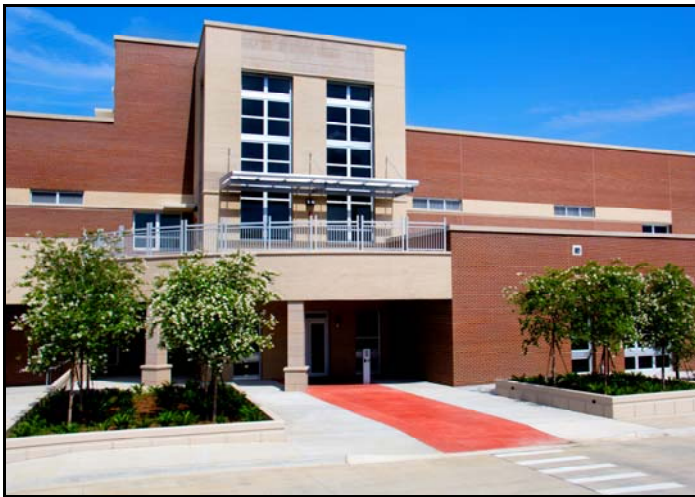
Public Safety Complex
