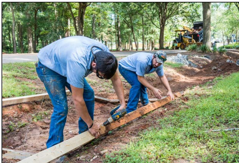
Construction of sidewalk for Community Safety & Mobility
