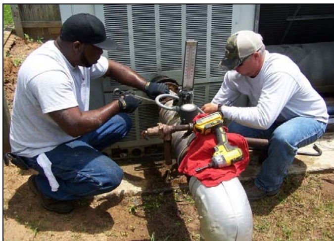
Building Mechanical Repairs and Improvements
