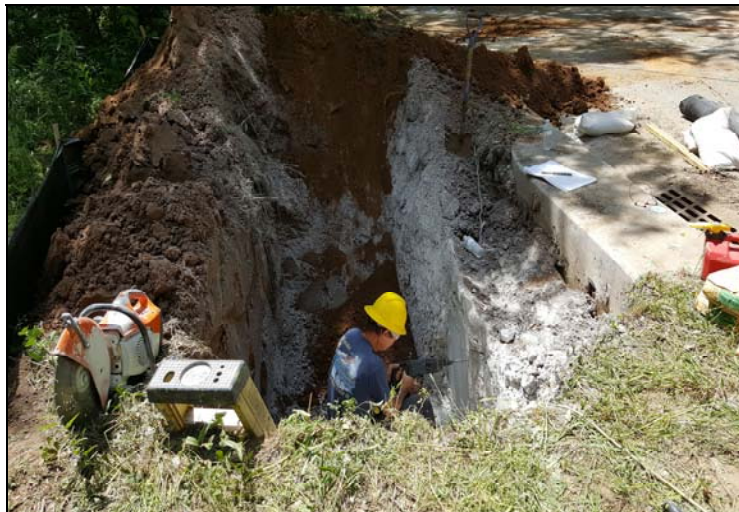
Stormwater Infrastructure Preventive Maintenance
