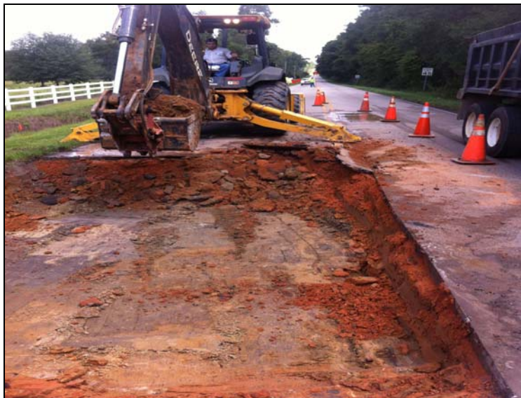
Asphalt Road Maintenance
