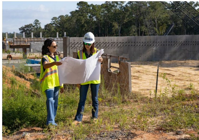
Northeast Gateway construction
