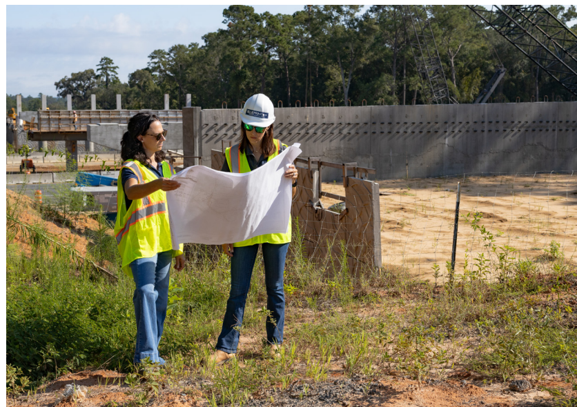
Northeast Gateway construction
