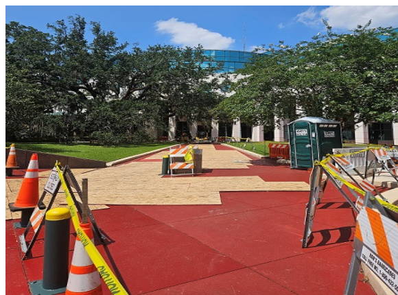
Building Infrastructure and Improvements - Courthouse Plumbing Repair
