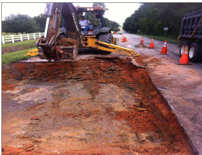
Asphalt Road Maintenance
