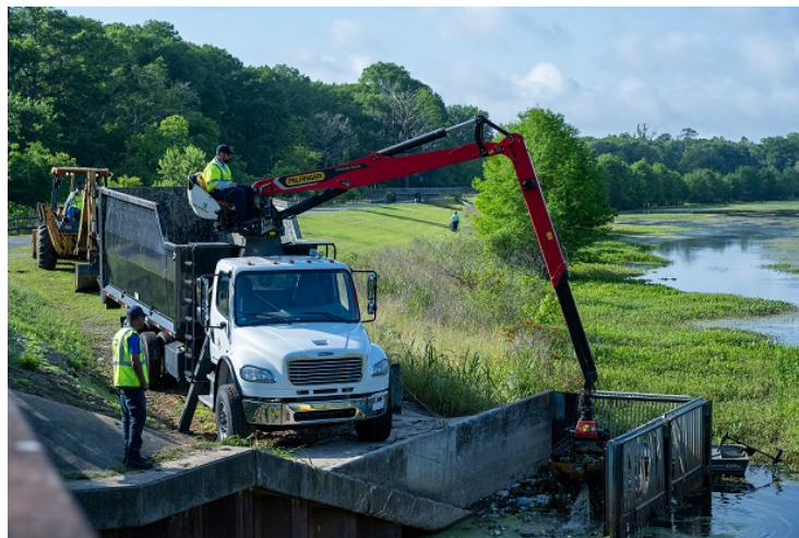
Stormwater Pond Repairs
