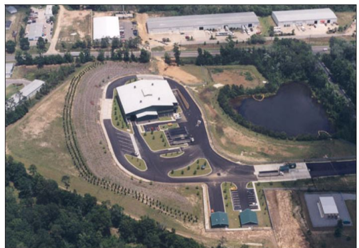
Leon County Transfer Station
