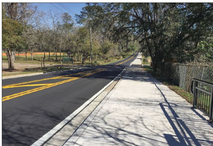
Local Road Resurfacing
