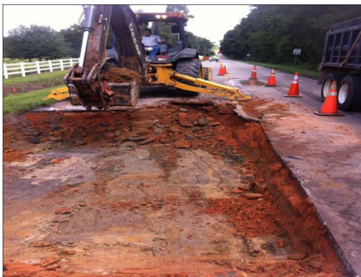
Asphalt Road Maintenance
