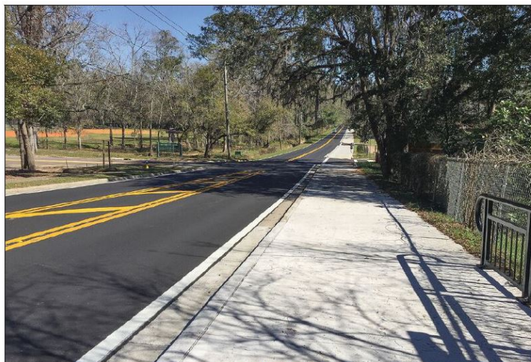
Local Road Resurfacing
