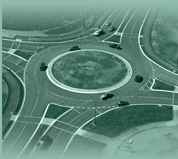
Over 5,000 roundabouts have been installed in Florida. Because of their safety and traffic calming features, roundabouts will continue to be an effective treatment and used in lieu of traffic signals or multi-way stop signs. Roundabout design features accommodate slower speeds while accommodating large vehicles like fire trucks and buses.
