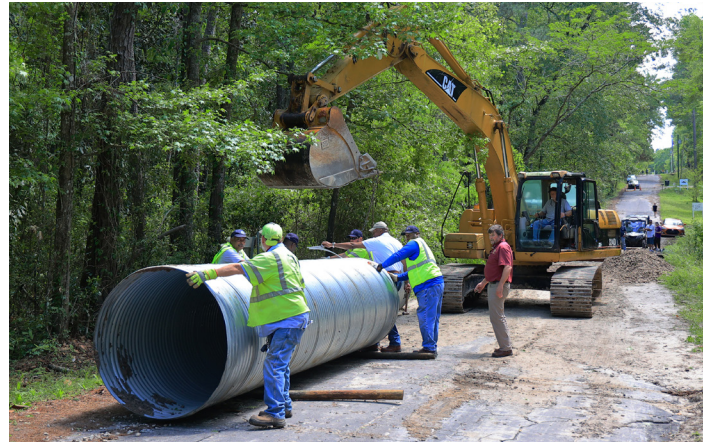
Sir Richard Road repair
