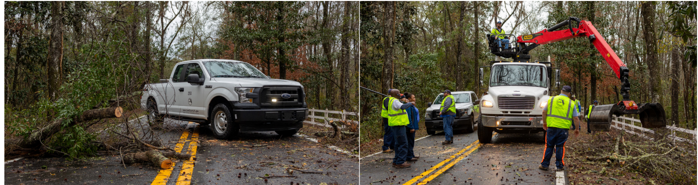
Clearing roadways after severe weather
