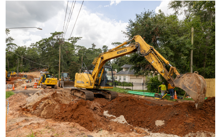
Magnolia Drive construction
