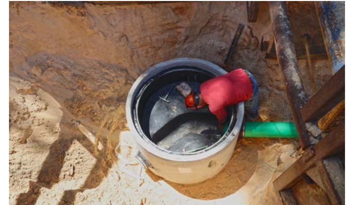
Septic to sewer construction
