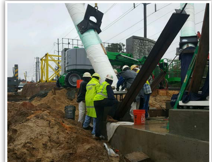
Bridge pier installation at Capital Cascades Crossing
