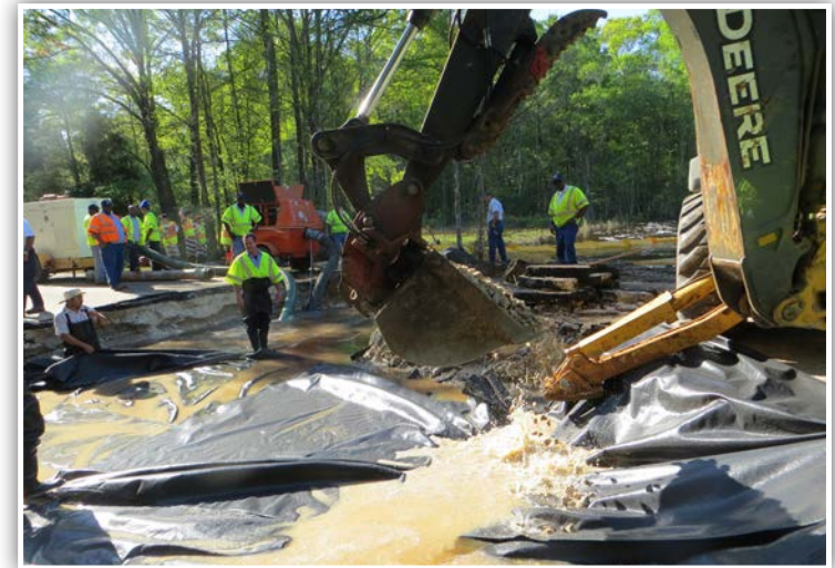
Repairing Tram Road
