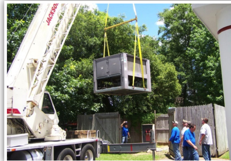
Loading Chiller at Dr. B.L. Perry, Jr. Branch Library
