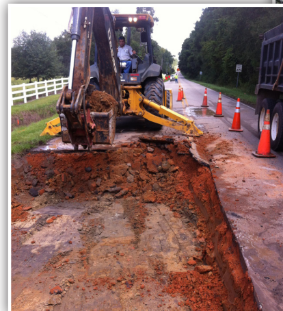
Asphalt Repair
