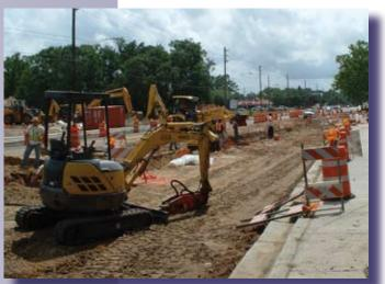
to Blair Stone Road and includes the following: roadway expansion from two to four lanes, landscaping, and the installation of sidewalks, bike lanes, curbs and gutters, and a stormwater drainage system.
