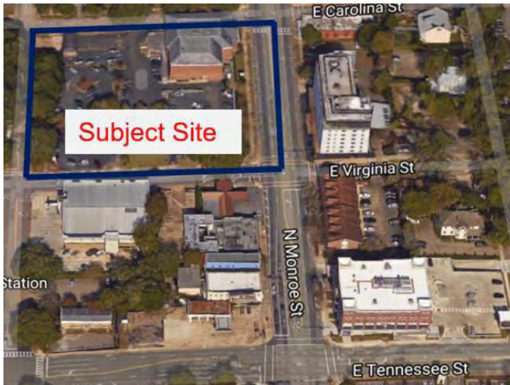
Aerial of Envision Credit Union site and surrounding properties
