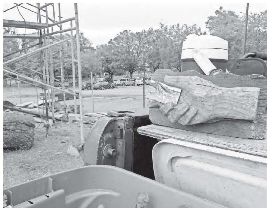
A carved hand at John Birch's job site at the library.
