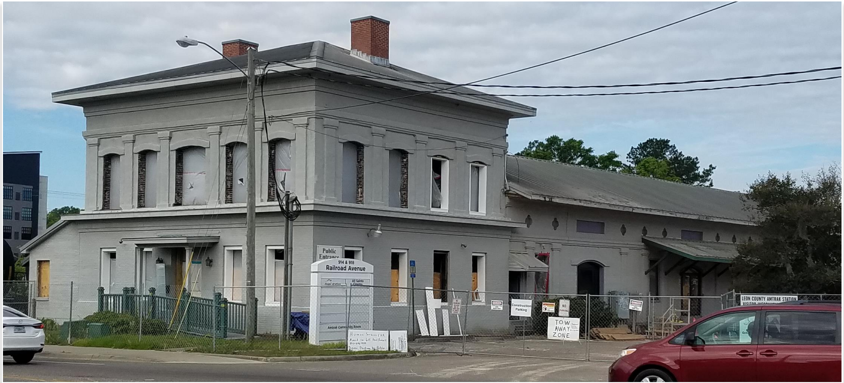
Northeast Corner - Office Area
