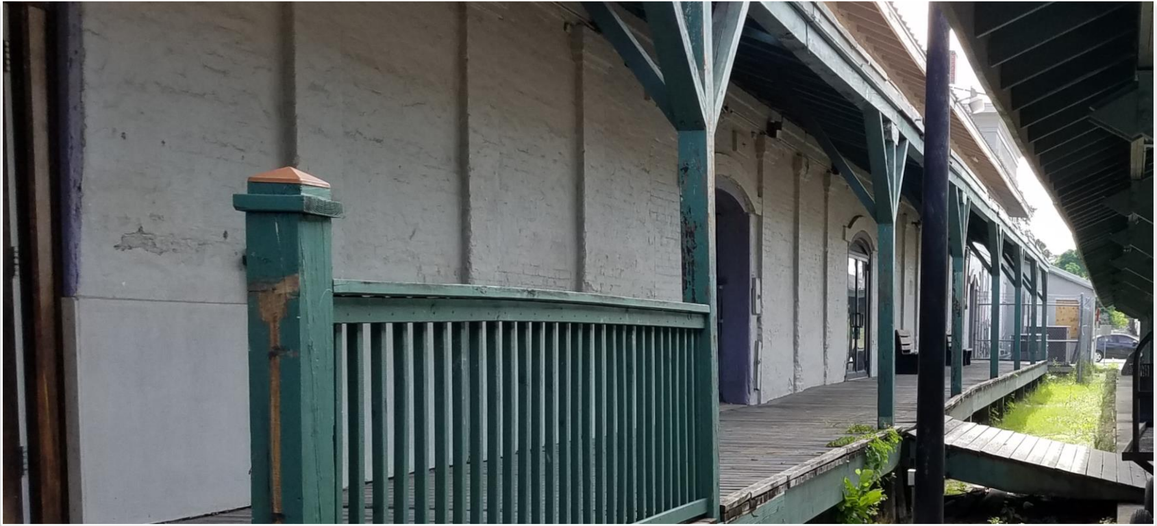
South Deck & Canopy
