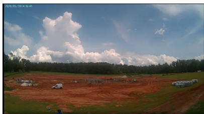
Construction of multi-use facilities at Apalachee Regional Park.
