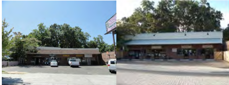
Gaines Street Square before the renovations (left) and after the renovations (right).
