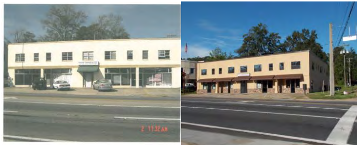
The Hinson Commercial Building before renovations (left) and after renovations (right).
