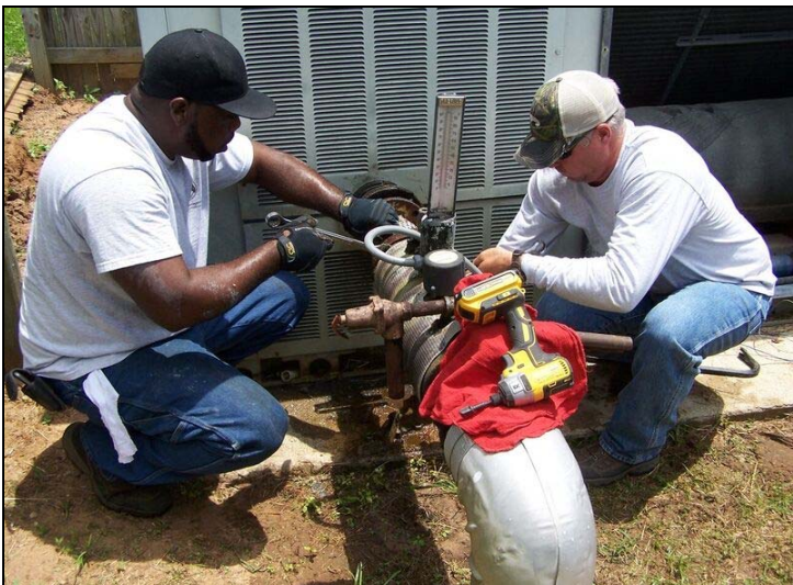
Building Mechanical Repairs and Improvements
