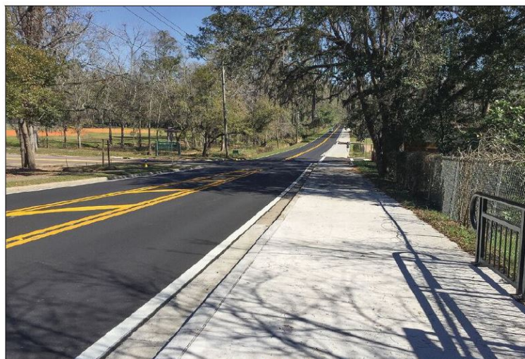
Local Road Resurfacing
