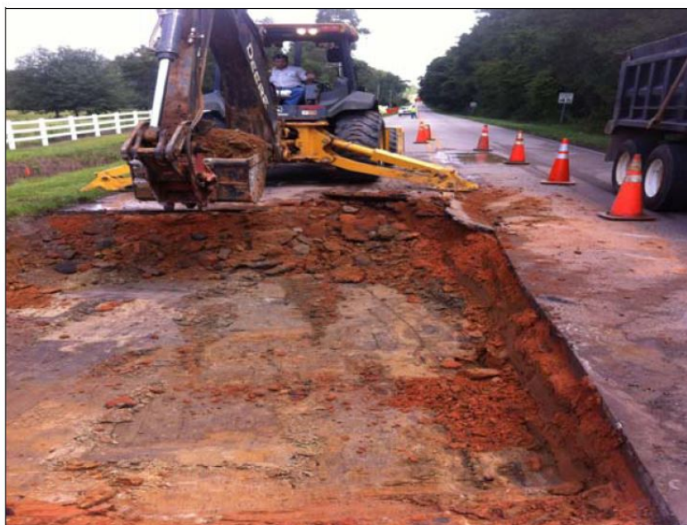
Asphalt Road Maintenance
