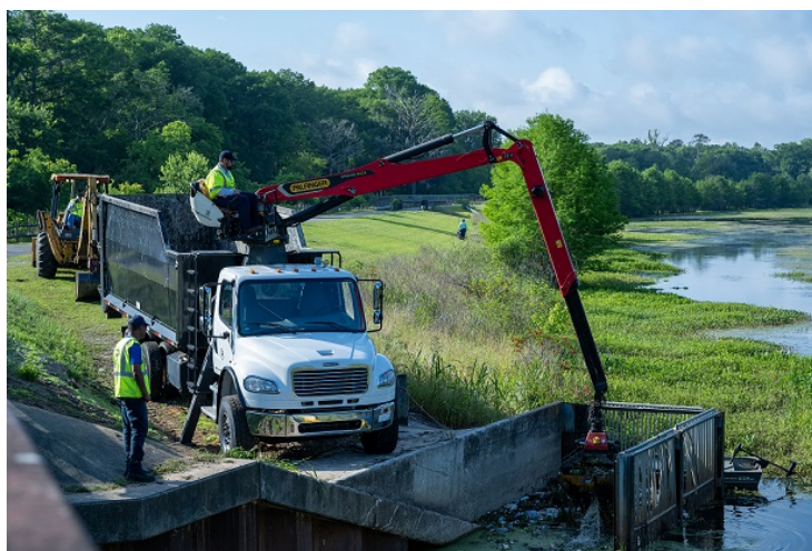
Stormwater Pond Repairs
