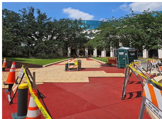
Building Infrastructure and Improvements - Courthouse Plumbing Repair
