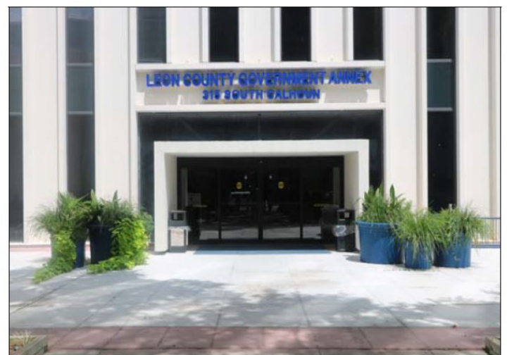
Leon County Government Annex Building
