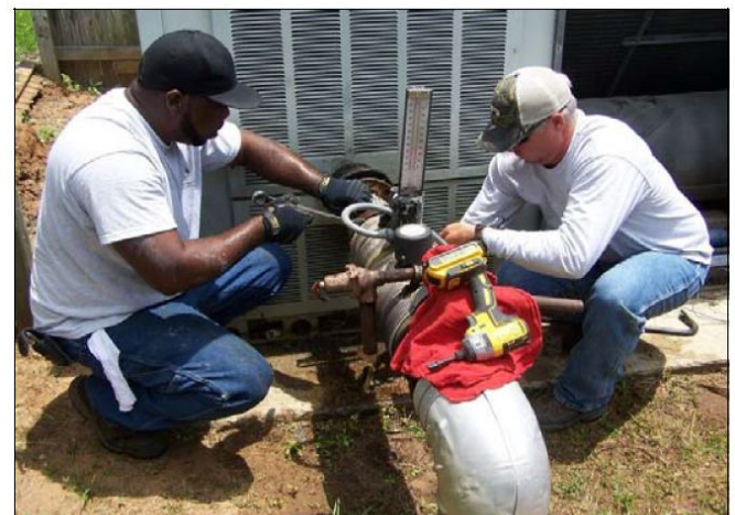
Building Mechanical Repairs and Improvements
