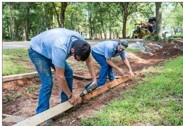
Construction of sidewalk for Community Safety & Mobility
