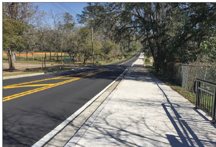
Local Road Resurfacing
