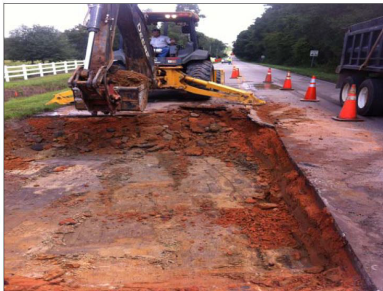
Asphalt Road Maintenance
