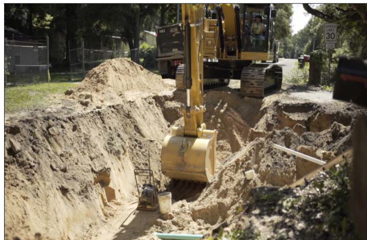
Stormwater Pond Repairs
