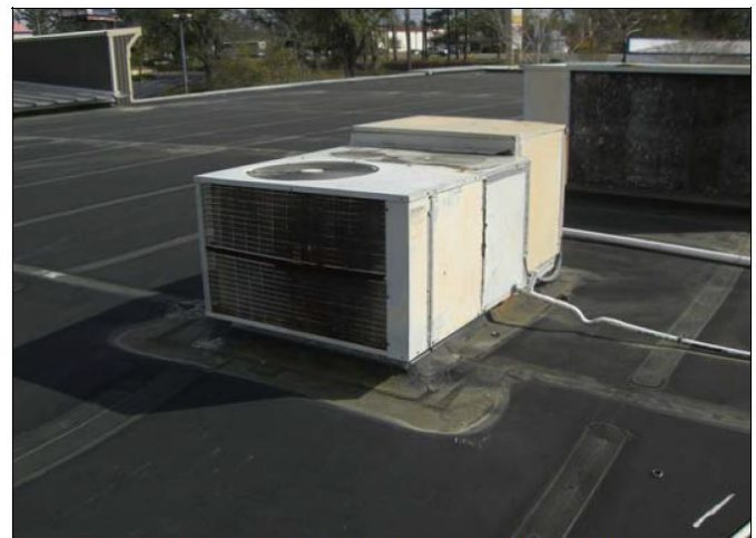
Building Roofing Repairs and Replacement
