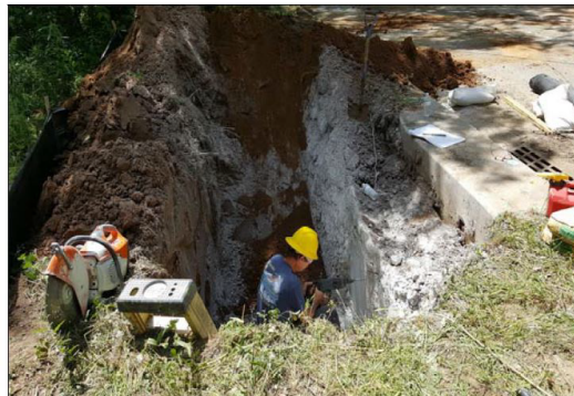
Stormwater Infrastructure Preventive Maintenance
