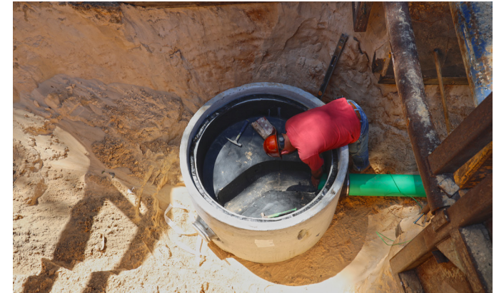
Septic to sewer construction
