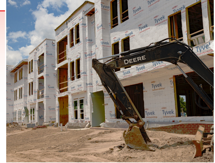
Orange Avenue redevelopment
