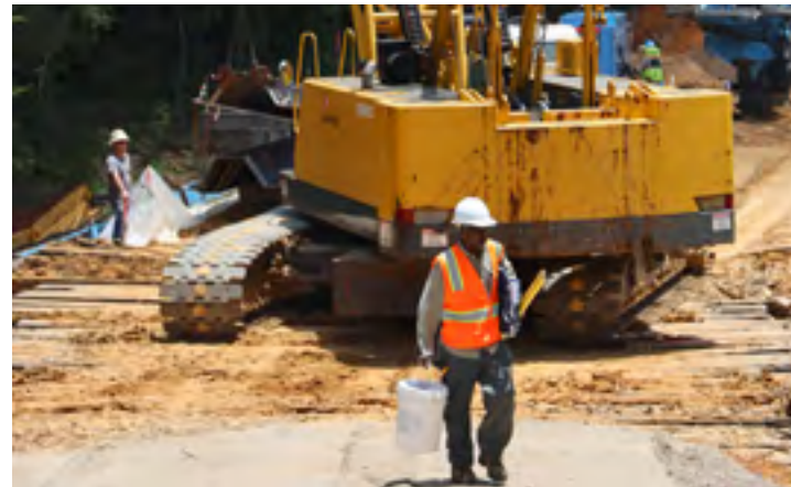
Centerville Trace Stormwater Improvements
