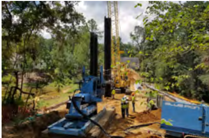
Centerville Trace Stormwater Improvements
