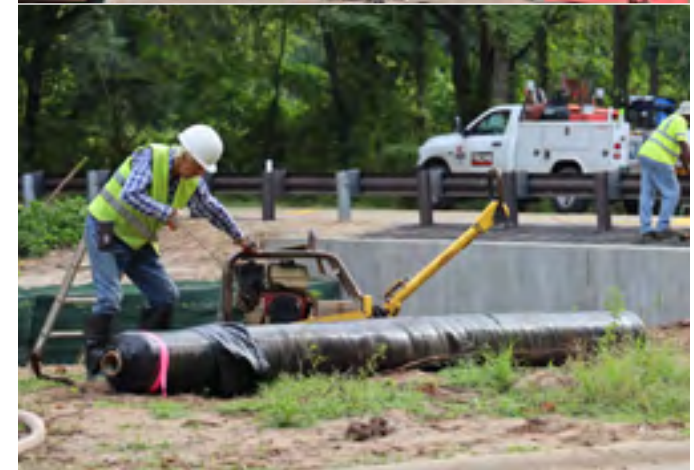
Meridian Road Drainage Improvements Project
