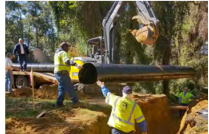
Crews place drainage pipe in Killlearn Lakes
