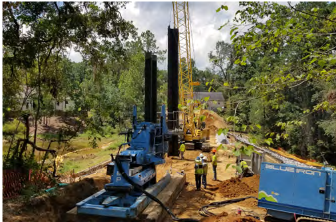
Centerville Trace Stormwater Improvements
