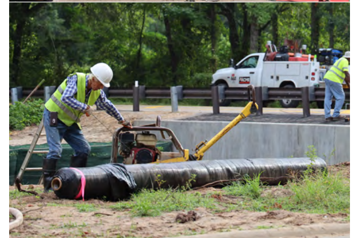
Meridian Road Drainage Improvements Project
