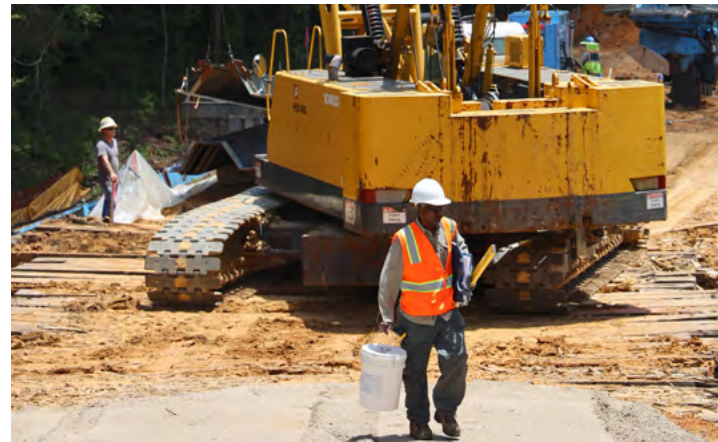
Centerville Trace Stormwater Improvements
