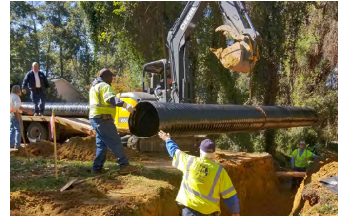
Crews place drainage pipe in Killearn Lakes
