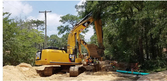
Woodside Heights sewer line construction
