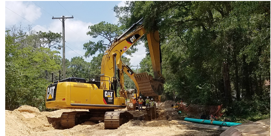
Woodside Heights sewer line construction
