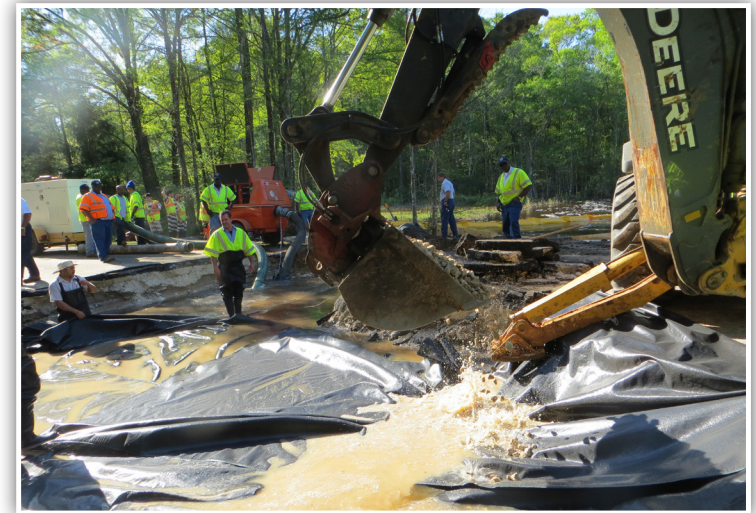
Repairing Tram Road
