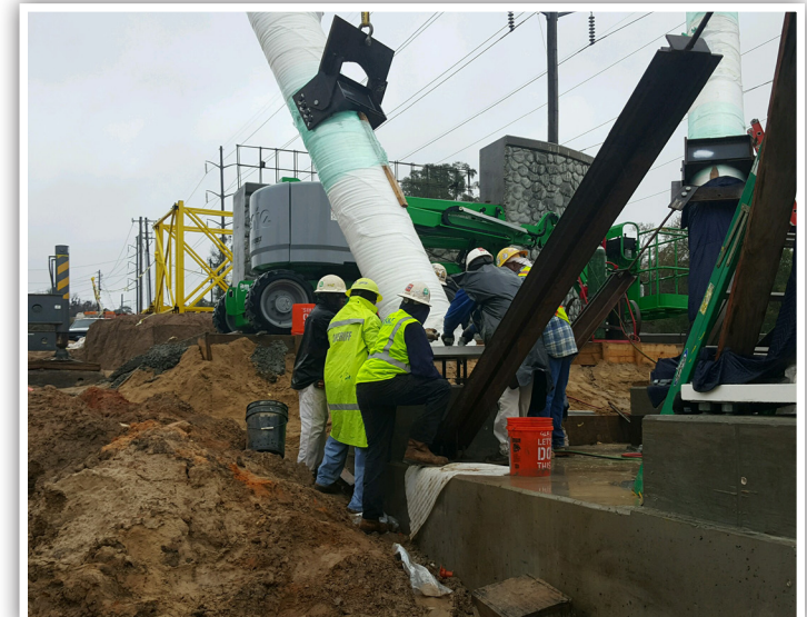
Bridge pier installation at Capital Cascades Crossing
