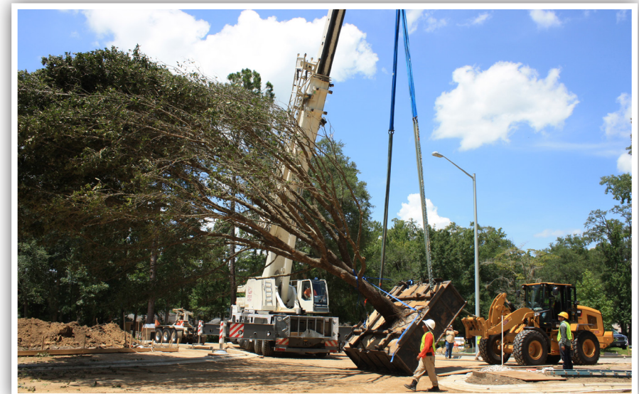
Planting of Live Oak tree at Kinhega Drive Roundabout
