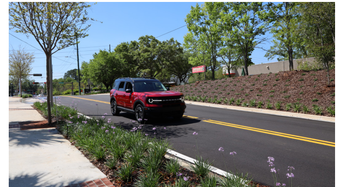
Major infrastructure improvements on Magnolia Drive
