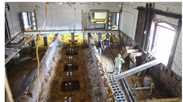
Renovations at Amtrak building
