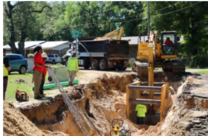
Annawood septic-to-sewer upgrades
