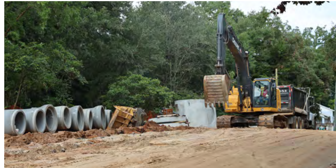
Major Infrastructure Improvements on S. Magnolia Drive
