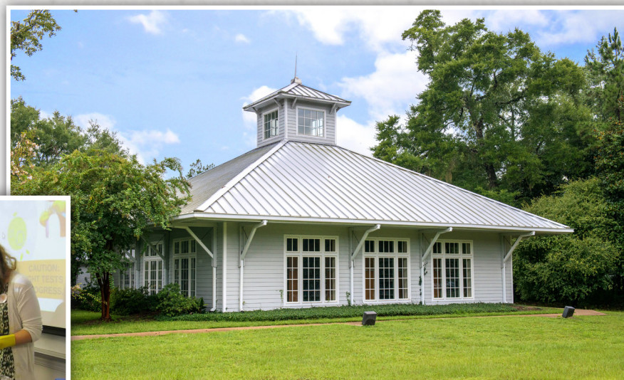
Fort Braden Branch Library
