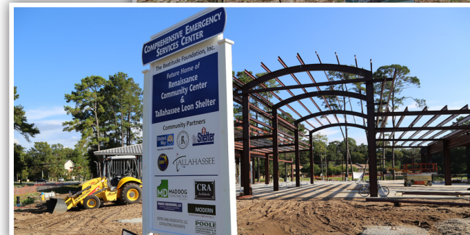
Construction of Comprehensive Emergency Services Center
