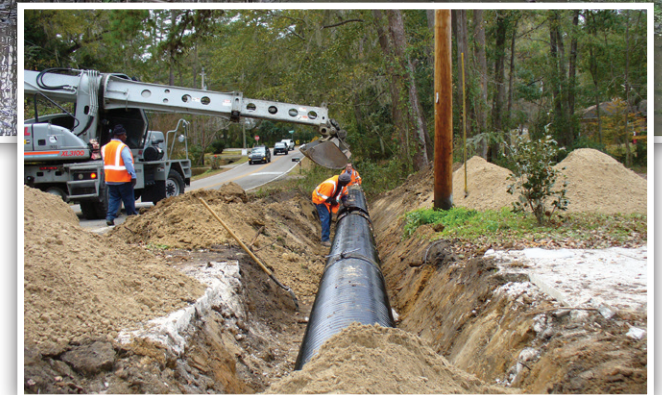
Stormwater crews installing driveway culverts
