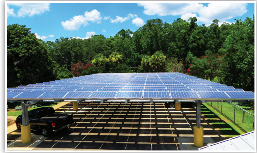
Cooperative Extension Net-Zero Facility
